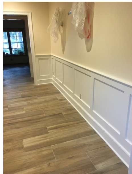
Figure 3 (finished PVC retrofit installation.)
