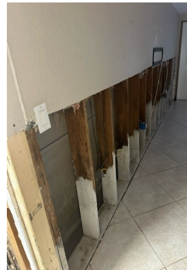
Figure 1. (4 foot drywall height removal.)
